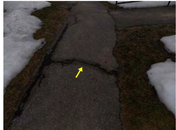
The site has asphalt-paved walkways. This is a close-up of a cracked section.
