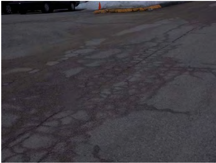
A close-up view of a parking lot section with cracks showing.
