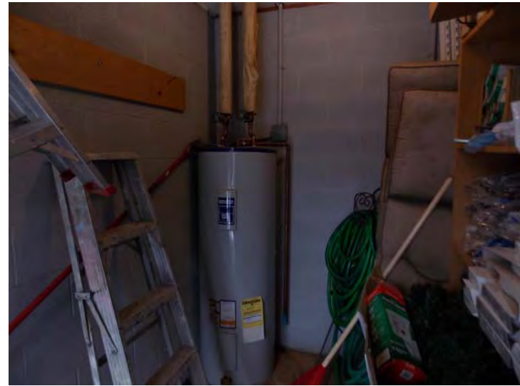
This is the electric-heated DHW tank in the community building.
