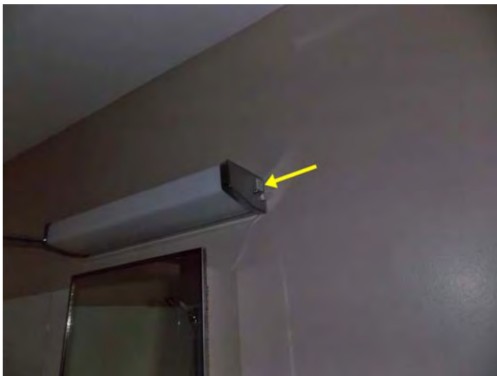
The only outlet in the bathrooms is the one off of the existing light fixture.
